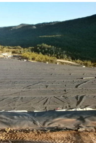
Final status of the temporary waterproofing work.
